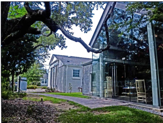
Fig. 26. WALTER ANDERSON MUSEUM OF ART, right, and OCEAN SPRINGS COMMUNITY CENTER, left, in downtown Ocean Springs. Because the buildings rest on the highest ground in the city, they escaped the floodwaters of Hurricane Katrina.
