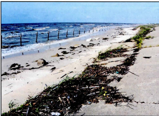
17. Beach/chenier erosion adjacent to Louisiana Hwy. 82 west of Holly Beach. This southern highway to Texas has had to be periodically moved inland into the marsh due to extensive erosion.
