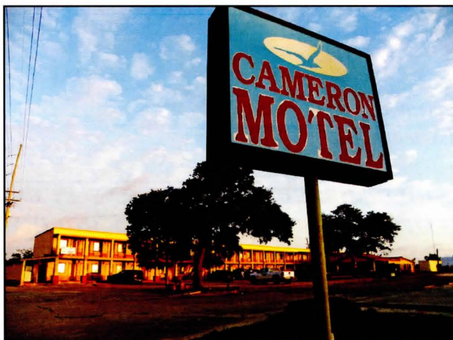
3. Renovated Cameron Motel in center of town. Although flood water reached the second floor during the latest hurricanes, the motel was renovated and is back in service.
