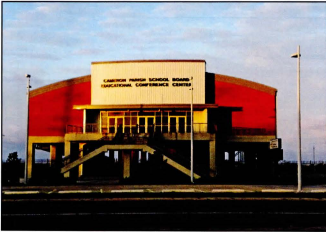
5. New Cameron Parish School Board Educational Conference Center across from the Cameron Motel. Current ordinances specify that all new construction be at least 12 feet above sea level.
